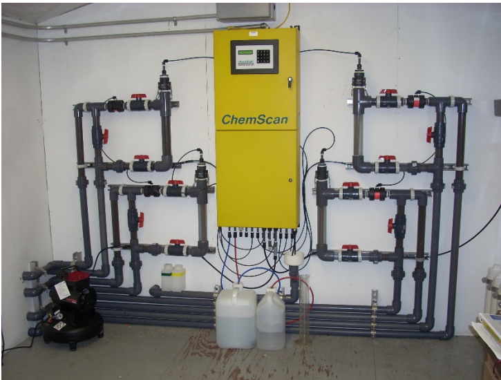
Single unit monitors up to eight sample lines at one time
