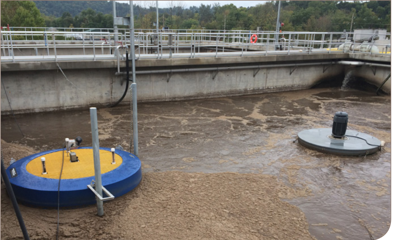
The patented floating decanter in the Alfa Laval AS-H Sequencing Batch Reactor System provides precise decanting for optimum effluent quality
