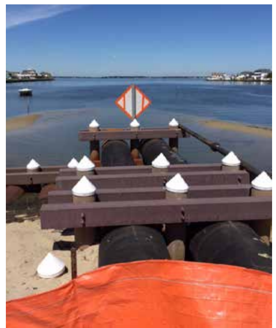
Drainage System pipes
