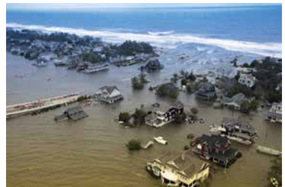
Route 35 devastation from Hurricane Sandy
