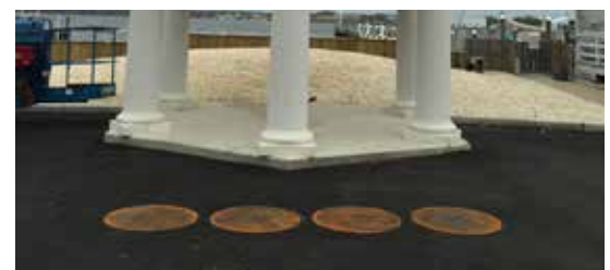
Completed view of a gazebo on Route 35
