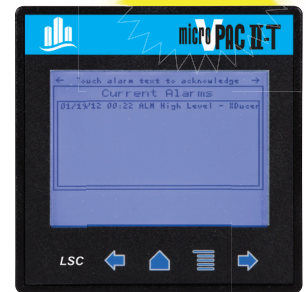
Current Alarm Screen
