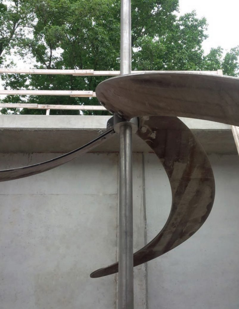
ARI 2 Anti-ragging impeller
