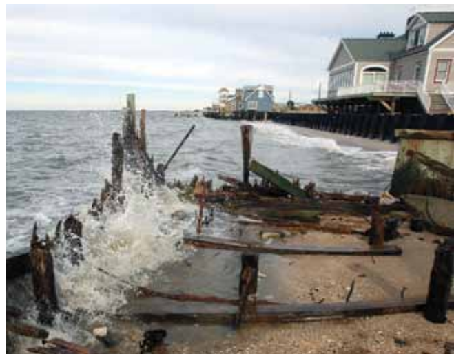
Aftermath of Hurricane Sandy's floodwaters
