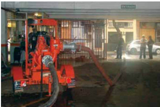
Godwin pumps dewatered approximately 30,000 cubic meters of water in Buenos Aires
